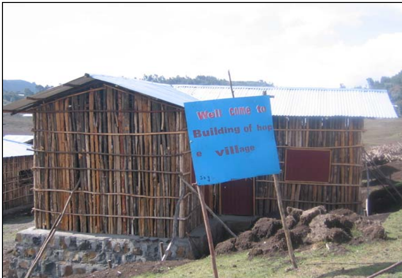
Unfinished 'chika' house (mud plastering)
